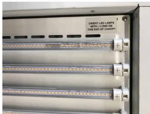
Figure 6-1 LED Tube Orientation
